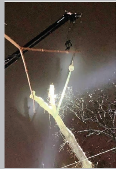
On December 4th in Vernon, we had to call in the help of IP&E Rigging to help remove large trees that had fallen on distribution lines feeding into Pleasant Valley Lake. Attempting to cut these trees would have damaged or broken the wire.
